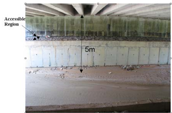
Figure 5: View from under the bridge
